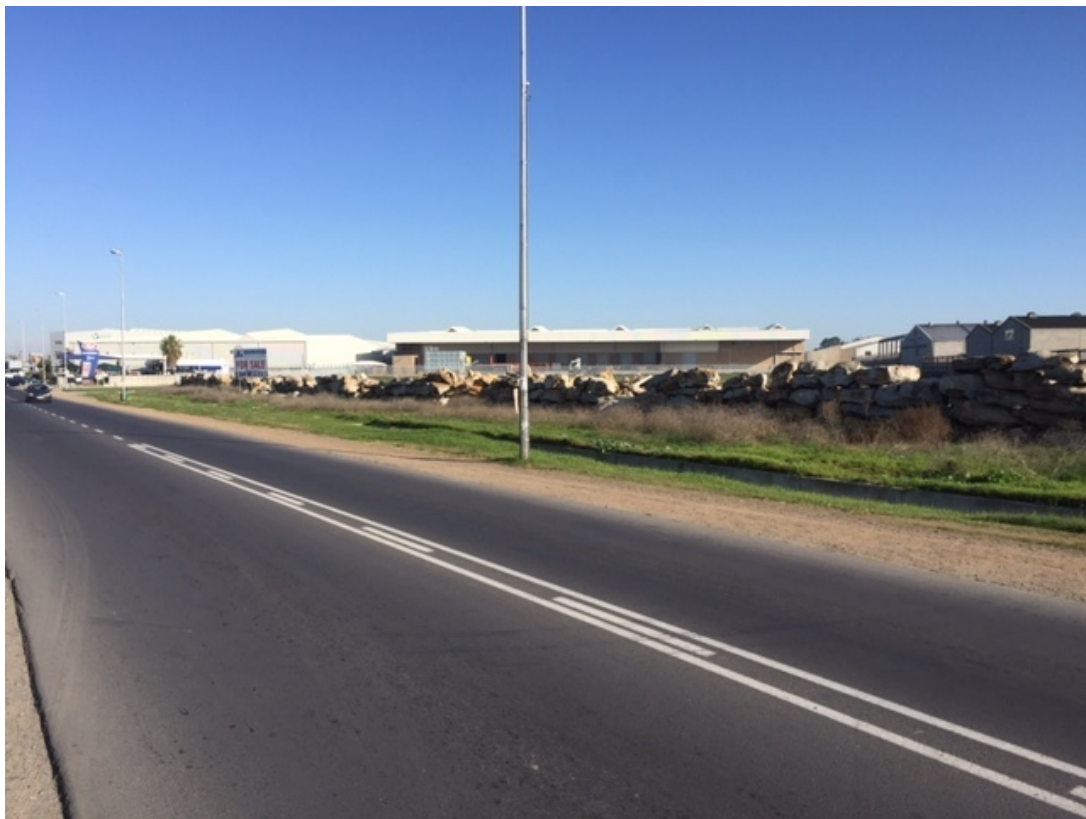
Before the project started
