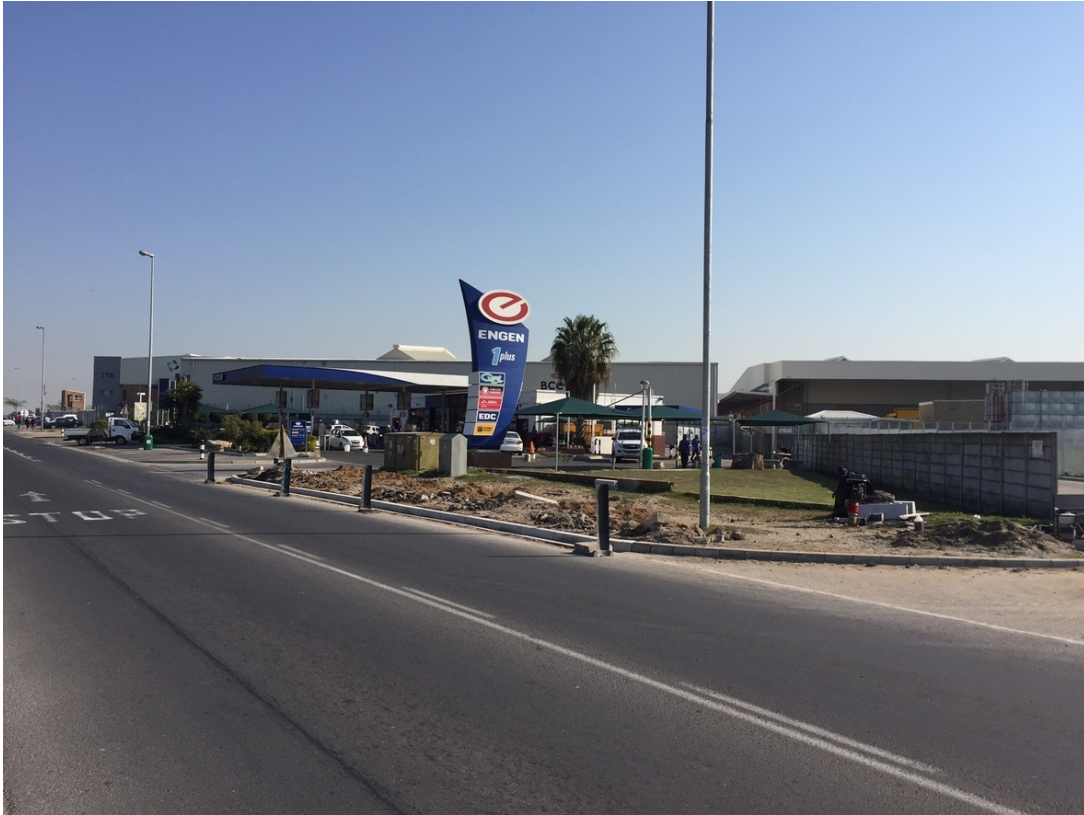
The upgrades near the Engen Garage
